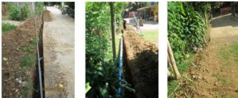
Expansion in Brgy. Village, City of Ilagan Isabela
