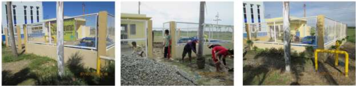
Improvement of City Terminal Pumping Station, Brgy. Alibagu, City of Ilagan, Isabela
